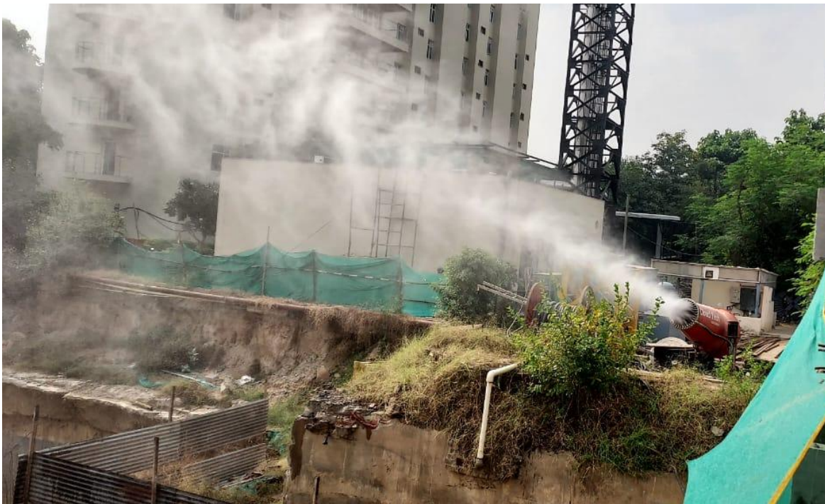
Photograph:- Anti-Smog Gun Installed at the Construction Site
