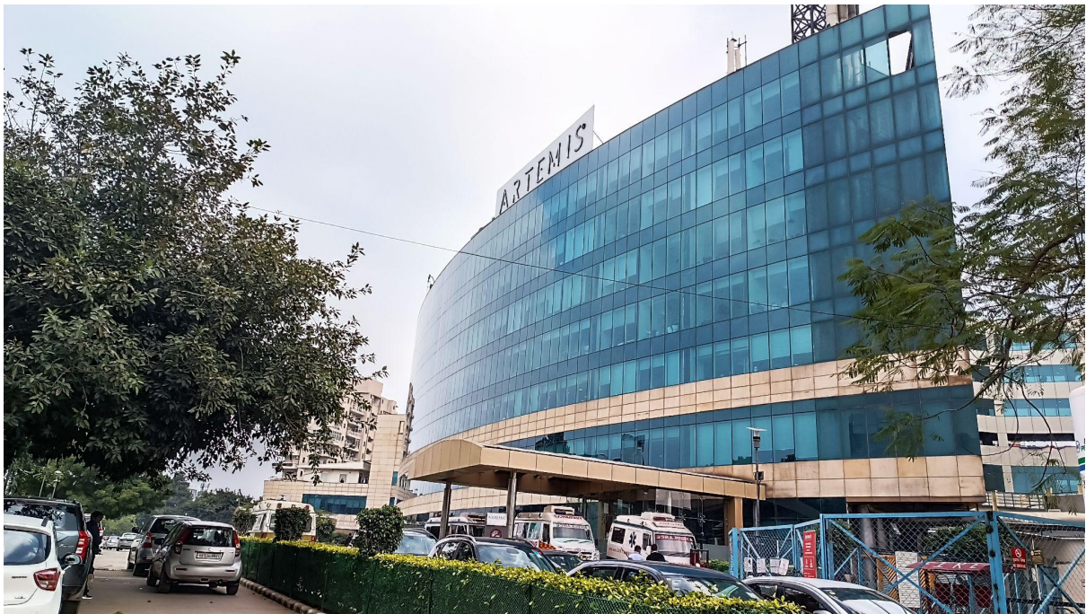
Photograph :- Operational Building
