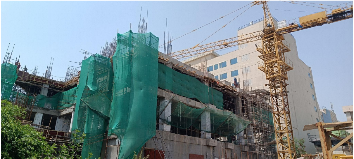
Photograph :- Under-Construction Building
